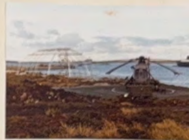
HANGAR BUILD AT NAVY POINT
