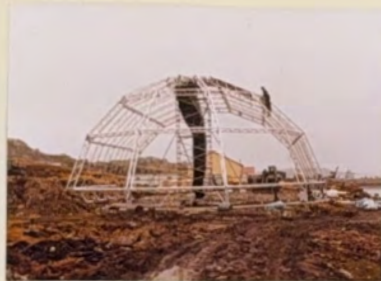
HANGAR BUILD AT NAVY POINT
