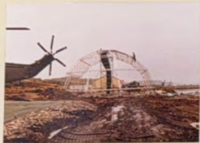
HANGAR BUILD AT NAVY POINT
