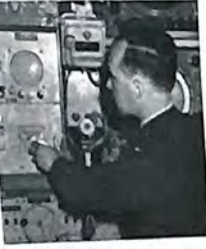
The course of the radio-sonde balloon is followed by radar in order to provide wind direction and wind speed at various heights
